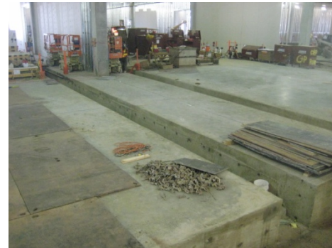
Figure 11 - View of the SOG with Trenches
