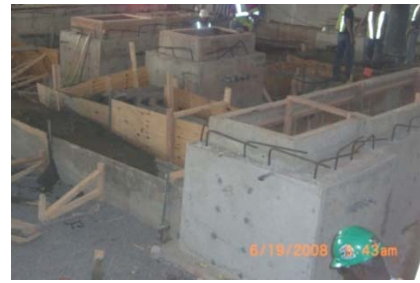
Figure 15 - Cast-in-place UPS pits
