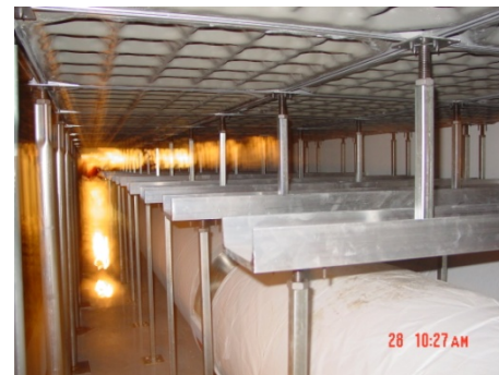
Figure 13 - Bridging over the chilled water pipes
